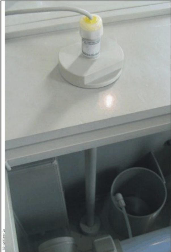
Level sensor with floater
