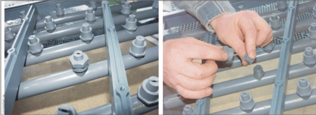
Inspection of spray nozzles
