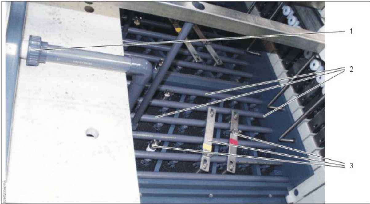
Supply cables removed from upper anode unit, pipe union still fixed
