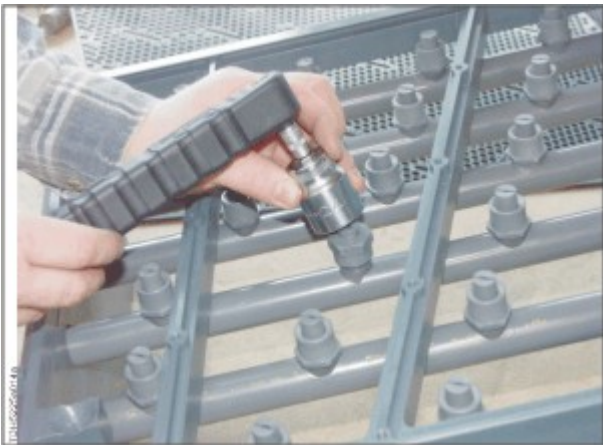
Reassembly of nozzles by a torque wrench (3 Nm)
